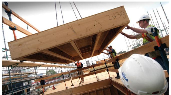
**B) LANDING OF A PREFABRICATED FLOOR CASSETTE**
